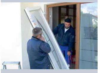
Step 2: The new Hörmann entrance door is fitted by the authorised Hörmann partner according to the measurements. The special entrance door threshold neatly covers up the transition from the interior to the exterior. The doors are fixed to the ground by concealed screws.
